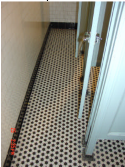
Picture 27- Men's Toilet Room B2
