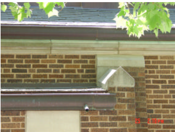
Photograph 3- North side showing gutters
