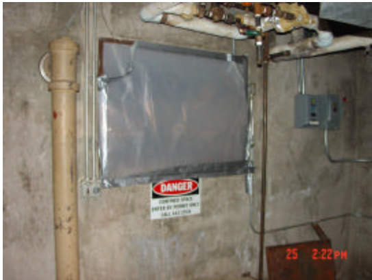
Picture 18- Hatch A to crawl space B8
