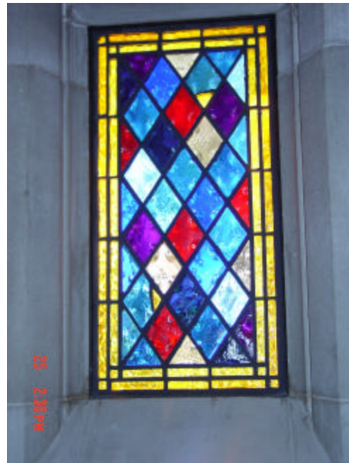
Photograph 11- South side "Dalle de Verre" interior
