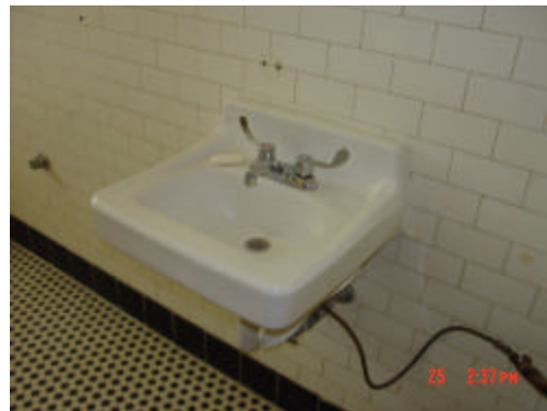
Picture 30- Women's Toilet Room 7
