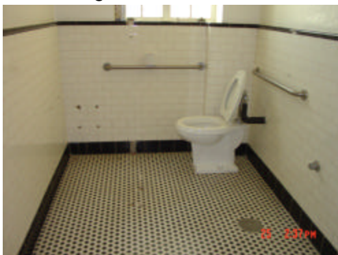
Picture 29- Women's Toilet Room 7
