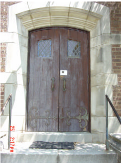
Photograph 12- Southwest Nave door
